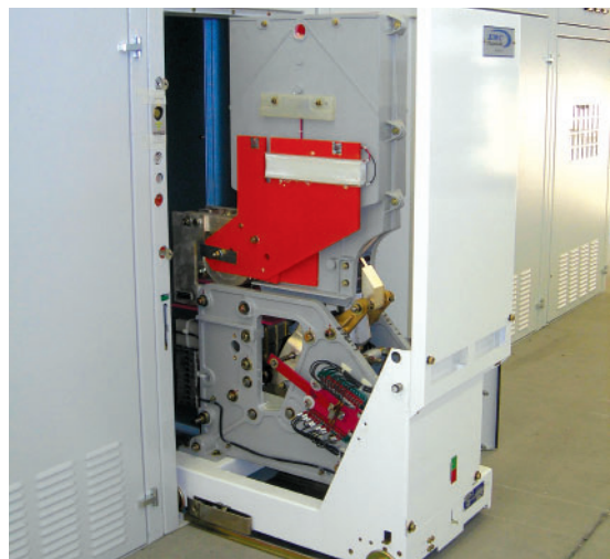
Feeder Cubicle
